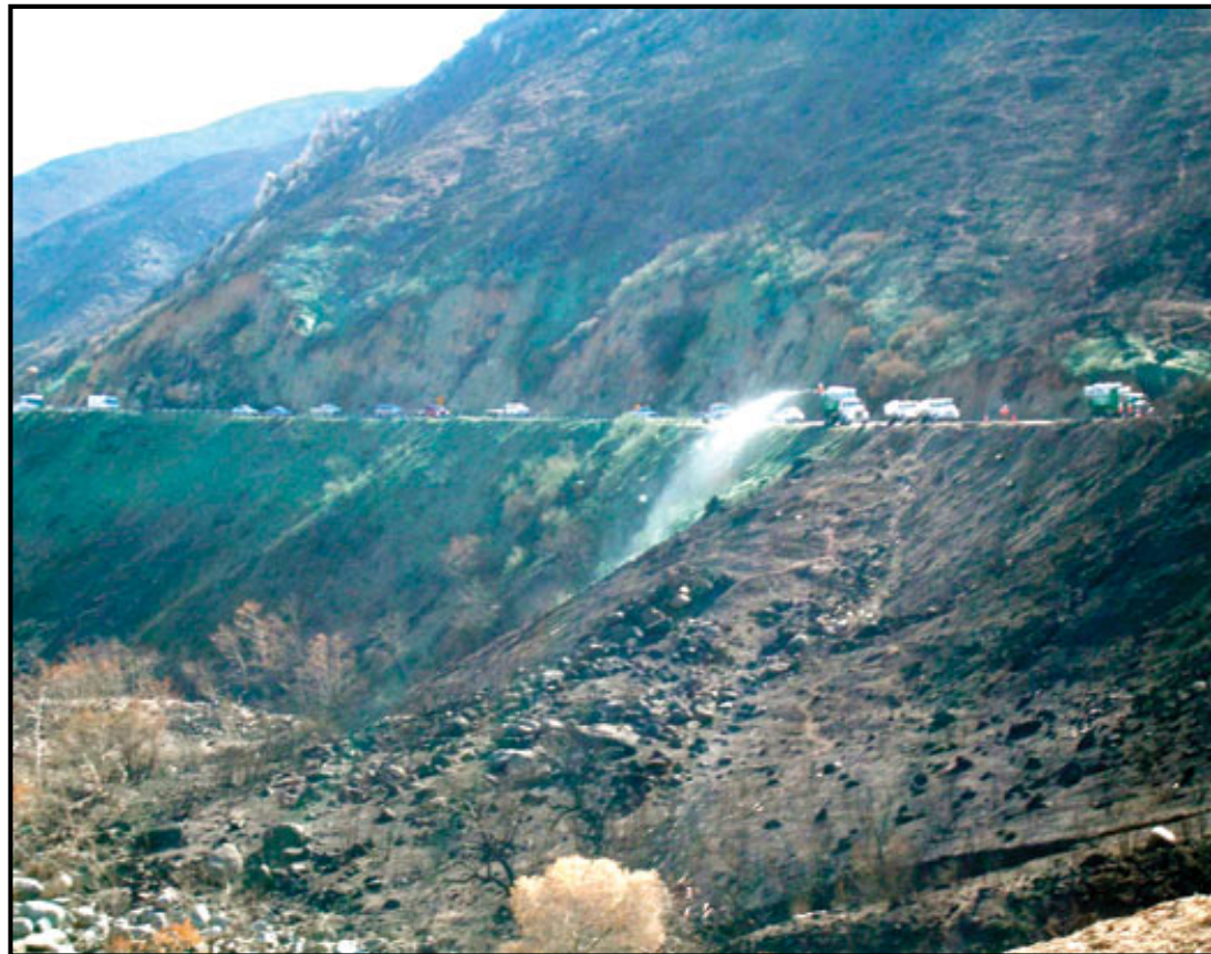
An example of the scale of the roadside areas treated.
