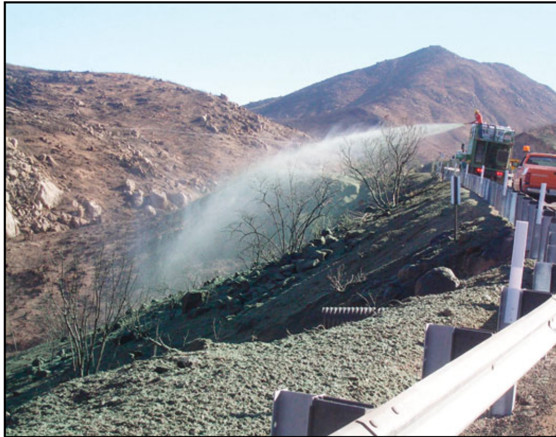
Hydroseed application of native nurse crop along I-15 in San Diego County.
